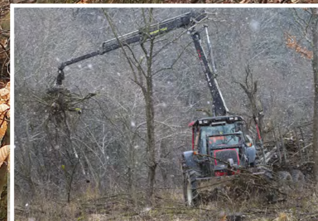
Clearing of cut trees and shrubs
